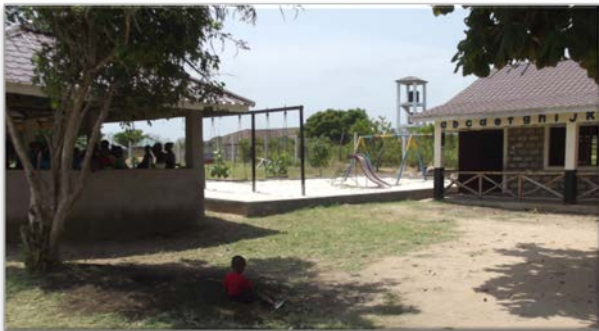
View of the new MAS Pre-School
